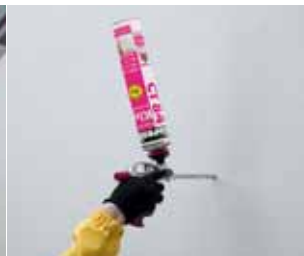
Filling in case of keying panels
