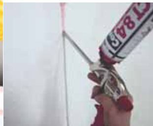
Filling in gaps between boards
