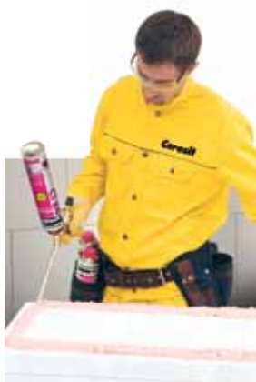
Fixing EPS board in thermal insulation system
